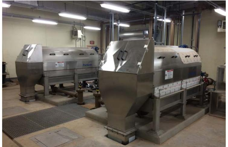
*Drum thickeners that produce filtrate high in BOD and ammonia*
