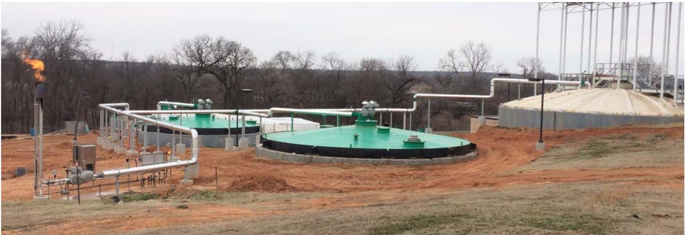
*Digesters where thickened sludge is transferred for anaerobic digestion*
