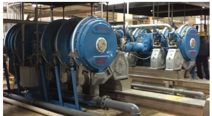
*Sludge presses that produce pressate high in BOD and ammonia*
